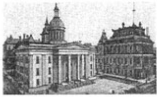
2nd Monroe County Courthouse by Merwin Austin, 1850
