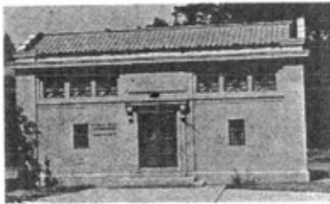
Cobbs Hill Gate House
