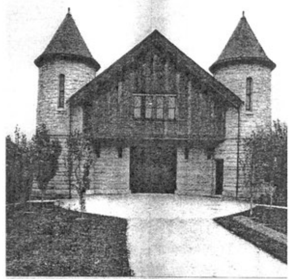
STABLES FOR G. E. EASTMAN, ESQ., ROCHESTER, N. Y. J. Foster Warner, Architect
