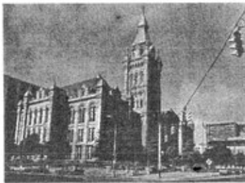
Eire County Municipal Building, 1871-75
